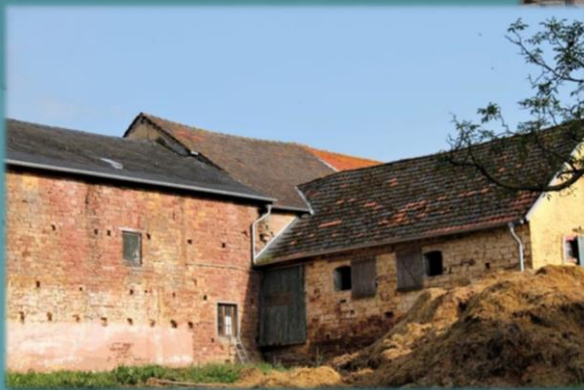
Figure 12-14 - Sievenicher Hof Farm 2018 – Red tiles after repair from crash
